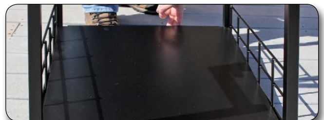
Figure D. Add the base plate on top of the bottom cross beams.
