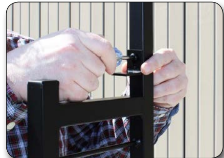
Figure C. Install the “L” brackets using the provided machine screws and nuts. Do not fully tighten the brackets to the frame.
