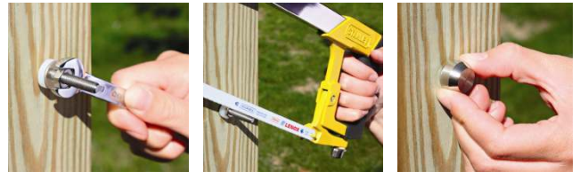
Figure M. The Deluxe Cover Nut Set installs in just 3 easy steps: tighten, cut and cover
