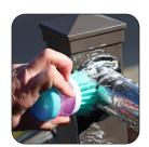
Scrub cable, fittings and framework (rails & posts) to clean off dirt, oils and contaminants
